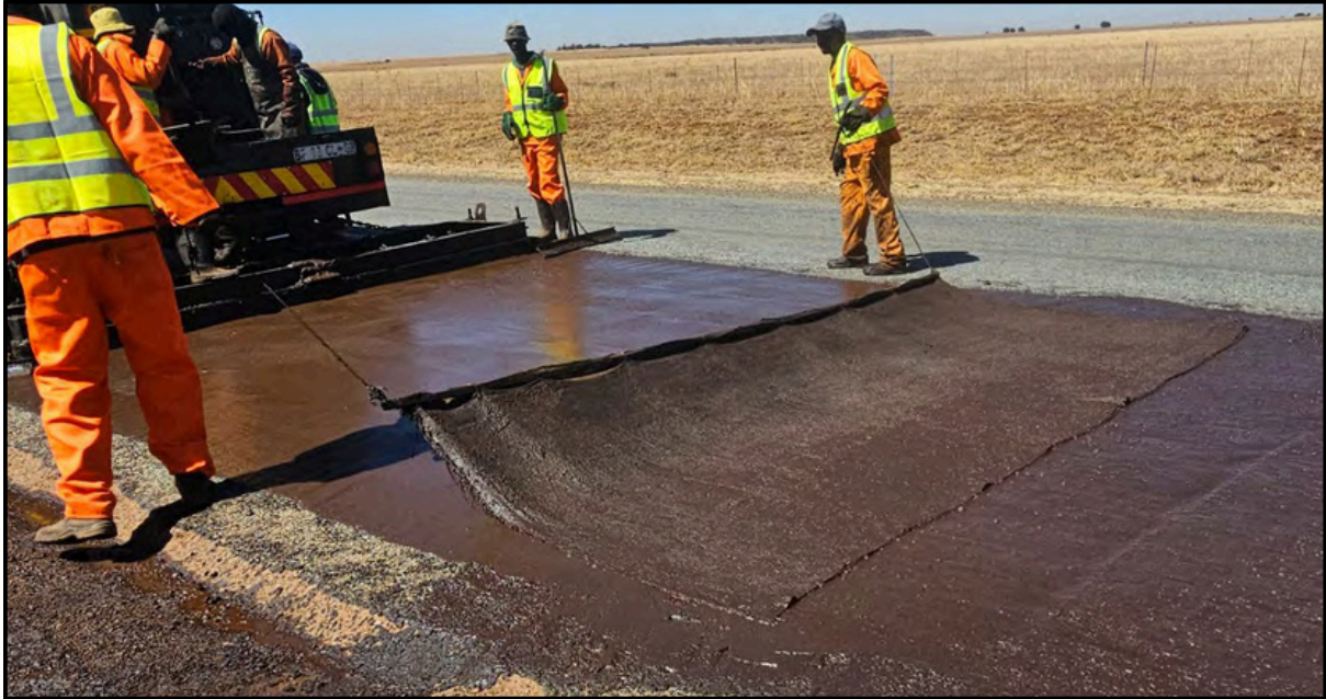
Figure 86 Application of a 12 mm MC-NME slurry using a continuous slurry machine
