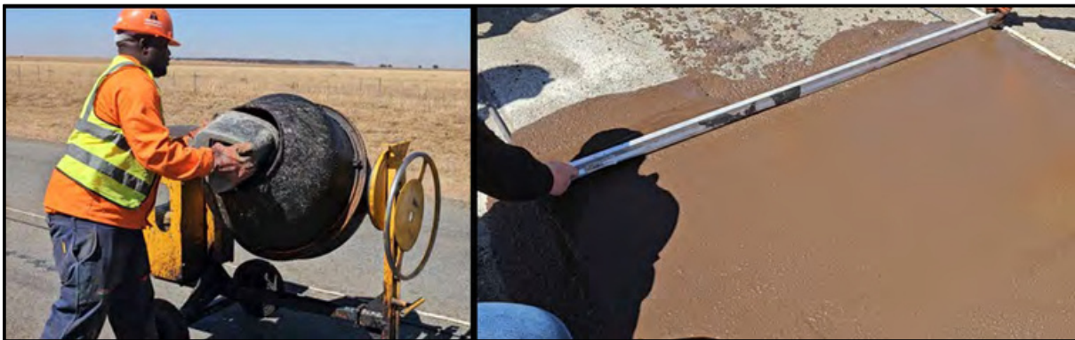
Figure 87 Mixing and hand application of a 12 mm MC-NME slurry
